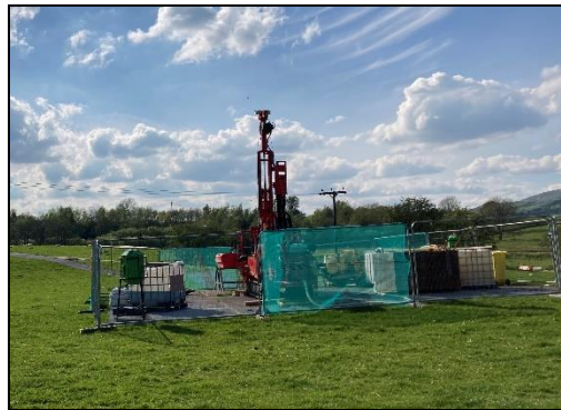
Typical GI survey working area
