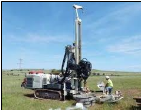
Sonic drilling rig
